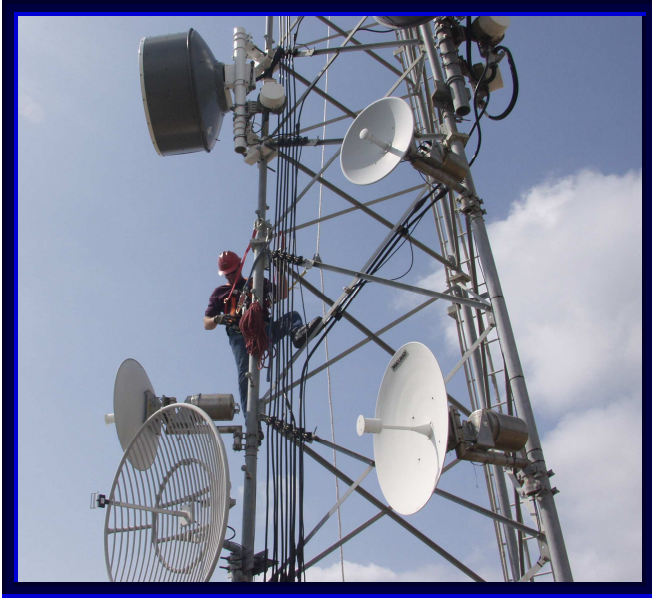
Ron Serabia, HPWREN, climbed the tower and installed wireless radios.
